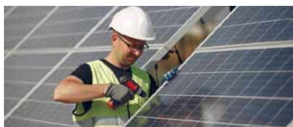
SOLAR SOLAR POWER
